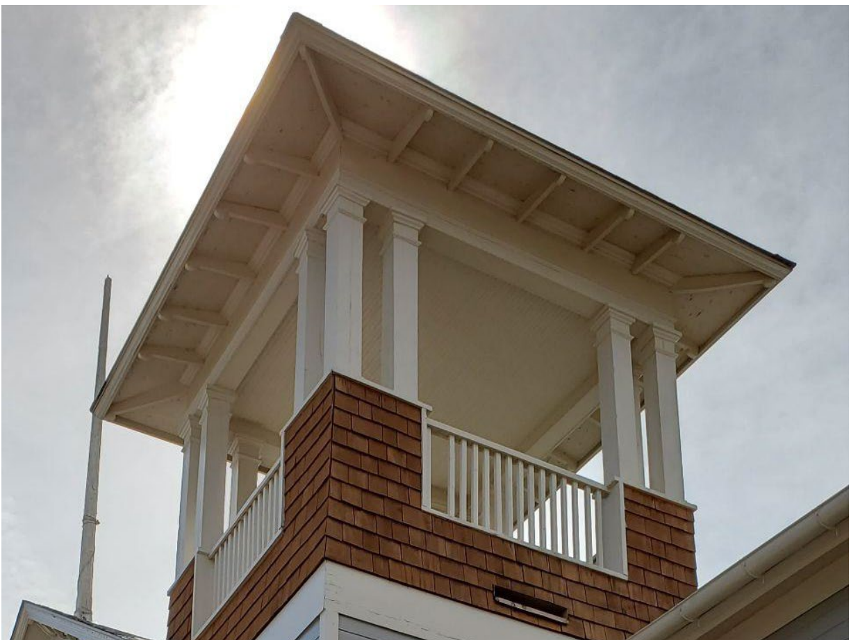
Figure 21: Chautauqua Dining Hall Tower, Exposed wood soffits with carved rafter tails (Lord, 2022)
