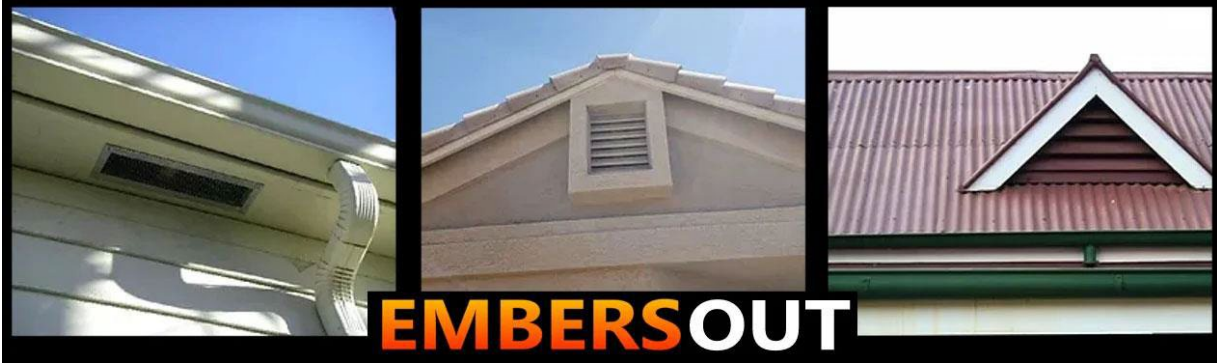
Figure 38: Photo from Embers Out Website of Retrofitted Vent Applications, Accessed May 22, 2023
