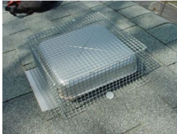
Figure 37: Roof Vent with Retrofitted Wire Mesh Cover (Roof Vent Screens Installation, 2023)
