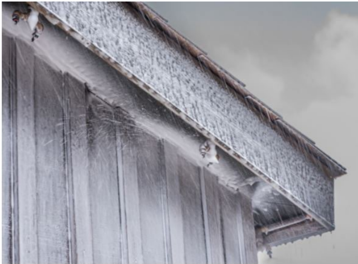
Figure 15: Defense System 2 Website Photo Soffit Sprinklers and Foam, Accessed May 23, 2023
