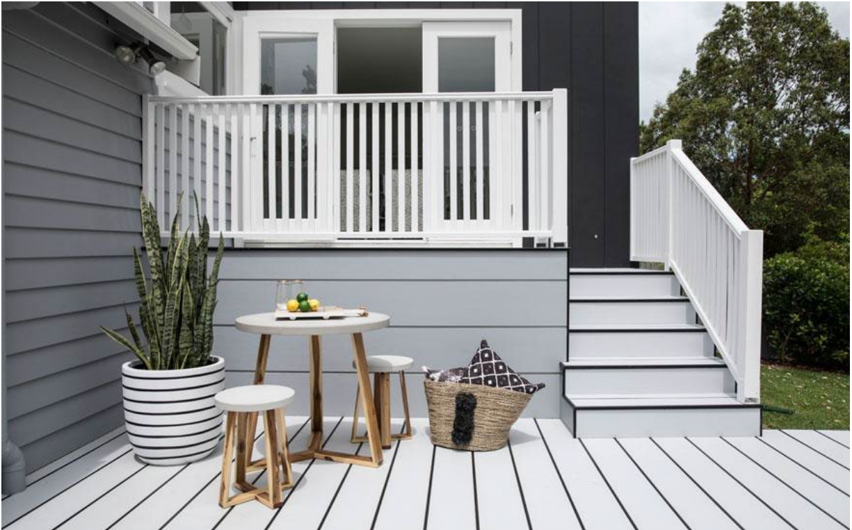
Figure 35: HardiDeck Website Project Photo, Accessed May 23, 2023
