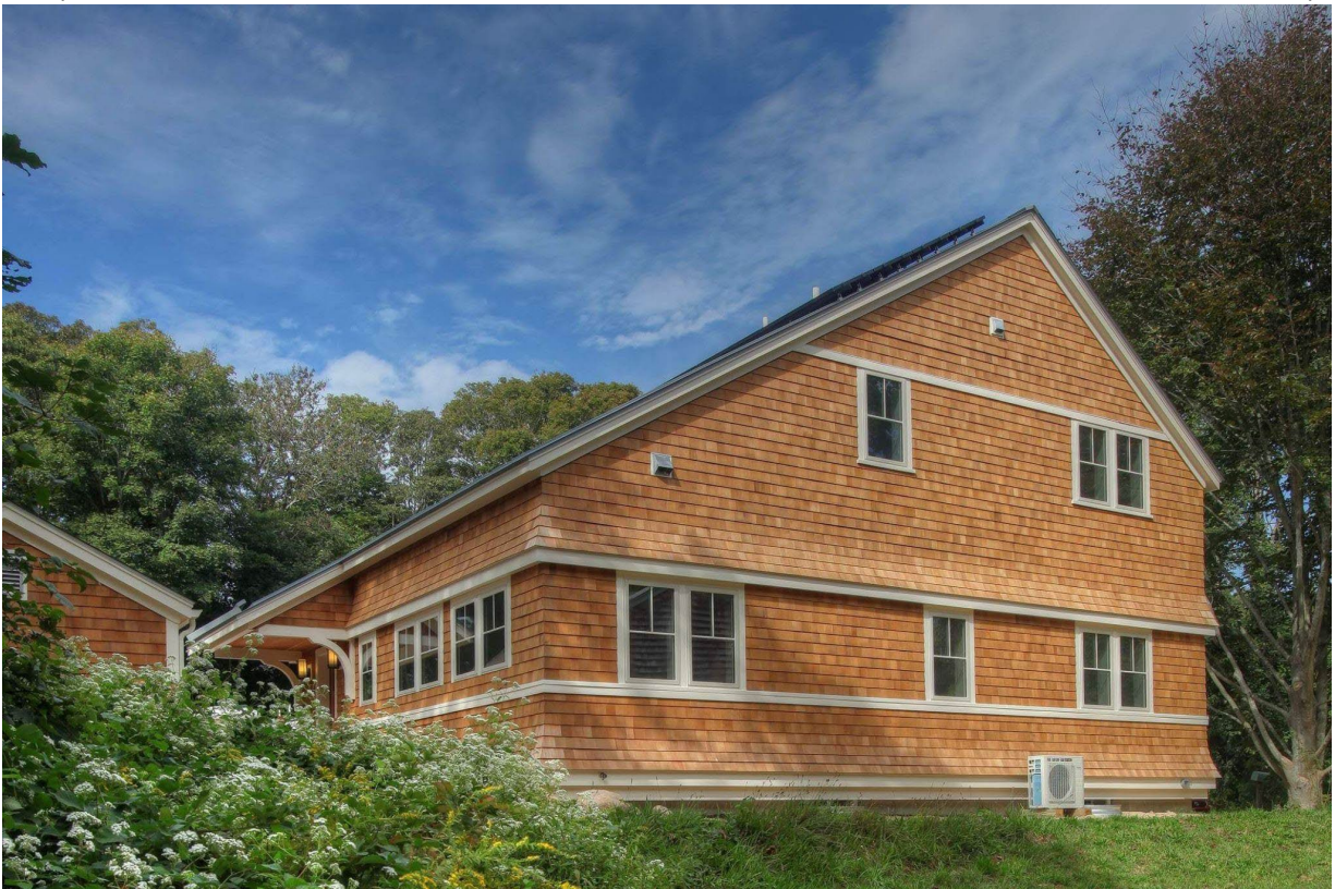
Figure 24: Cedar Valley Website Photo, Custom Massachusetts Home Installation, Accessed May 22, 2023
